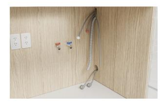
**12.** Route the power cables and hoses through service holes.
