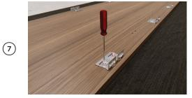
Secure the side brackets using two screws per bracket. Ensure side brackets are fitted tightly and the fasteners are secured straight.
