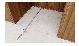
Measure the depth range of the alcove ensuring the minimum depth range has been met.
