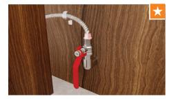
Connect to tap and turn on. If water is running, check for leaks.
