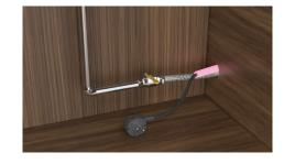
Route the hard wiring through the service hole in the side of the cabinetry. Tape to the floor to secure.
