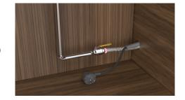
Briefly turn on the water supply and check for leaks, once you are satisfied the connections will not leak turn off the water supply.
