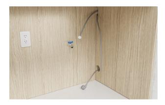
8. Route the power cables and hoses through service holes. Ensure power will remain accessible following install to allow access for any future product maintenance.
