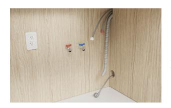
**5.** Route the power cables and hoses through service holes. Ensure power will remain accessible following install to allow access for any future product maintenance.
