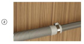
Pull the hose through the drain hose support before threading the hose clamp onto the hose and fitting to the sink trap. Secure to trap using the clamp. Ensure hose is routed straight to the trap.
