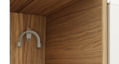
Install the drain hose support to the back wall, as close to the underside of the countertop as possible. Refer to 'Plumbing & electrical considerations' for minimum install heights.
