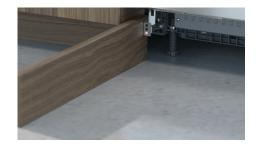
Mark the pilot hole locations for each bracket. Measure the centre of the panel and mark 237mm to each side. To determine the height of the brackets, measure the height of the lowest bracket hole against the toe kick panel.
