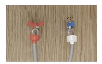
**9.** Connect the cold hose to cold water tap and turn tap on.
