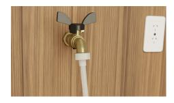
Ensure the rubber washer is fitted to the coupling before connecting the inlet hose to the tap. Hand-tighten into place.
