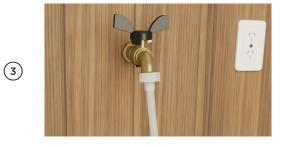
Ensure the rubber washer is fitted to the coupling before connecting the inlet hose to the tap. Hand-tighten into place.
