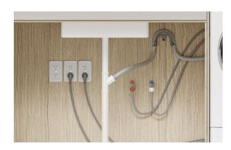
**16.** Connect the power cables and check products are powered on and are connected.
